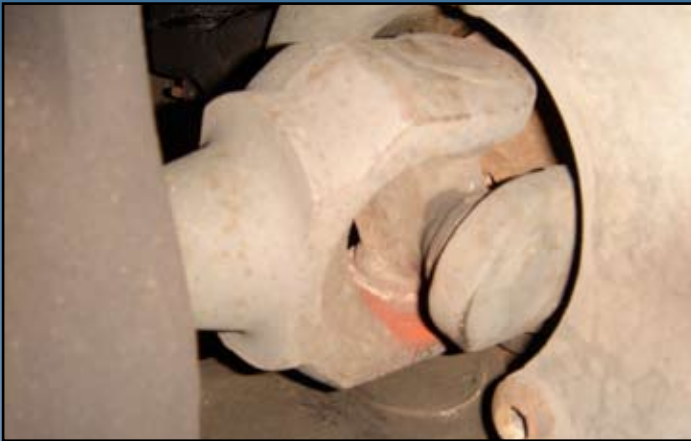
Rust dust evident around the axle universal joint
